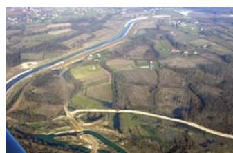
An aerial view of the Gomjenica river diverted from its course to accommodate the Buvac mine. Photo by Miso Danicic, Eko Pokret Omarska
