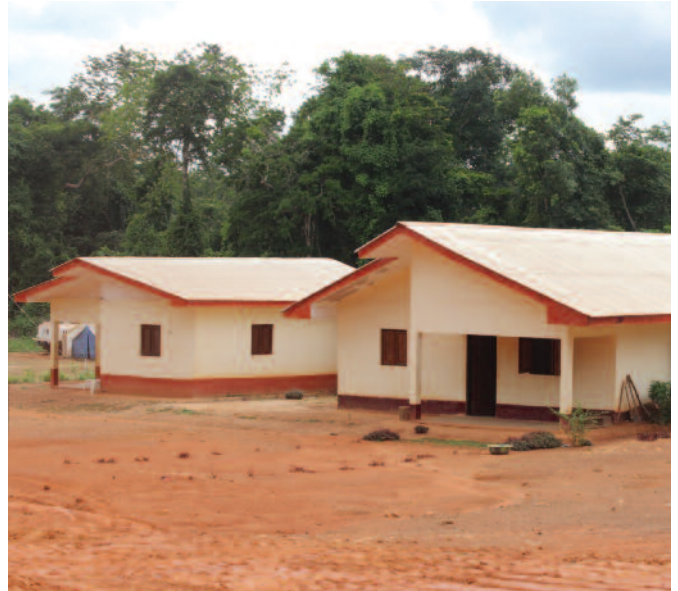
Concrete Structure Built by PIOM for Community Member Resettled from Airstrip Facility, Grand Gedeh County. © SDI
